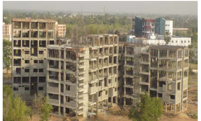
Boys Hostel (Capacity: 450 capacity) 45% complete (RCC of 6 th and 7 th floor is in progress)
