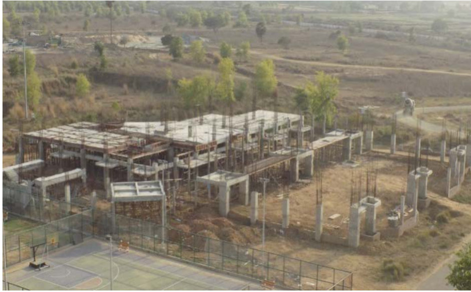
Gymkhana: 35% complete (RCC work is in progress)
